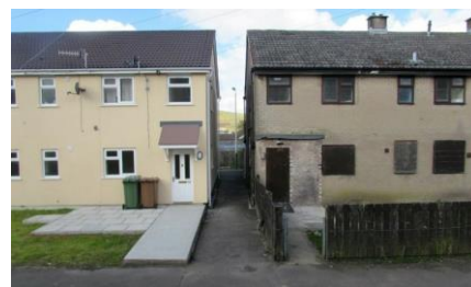
63 - WHQS external improvements
