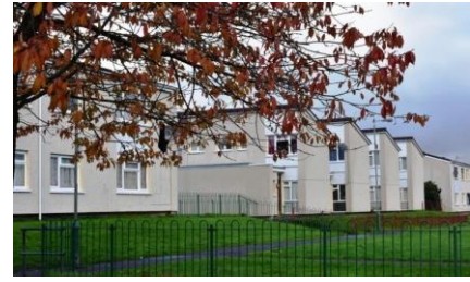
66 - WHQS external improvements at Lansbury Park
