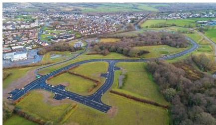
71 - New road network at Tŷ Du mixed use site, Nelson
