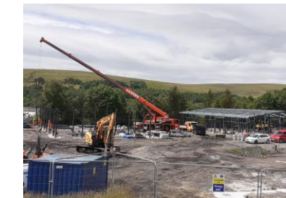
75 - Works at the Lawn Industrial Estate, Rhymney
