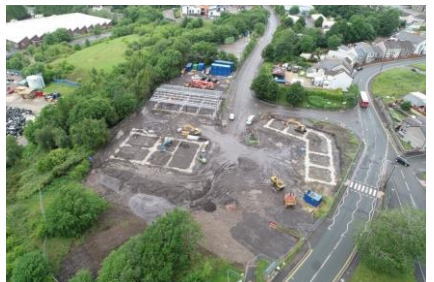
74 - Works at the Lawn Industrial Estate, Rhymney
